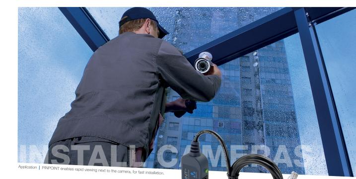
Focus and adjust IP cameras with PINPOINT quickly and easily
